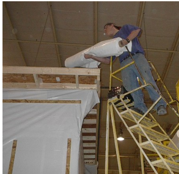
Figure 54 Lifting a roll onto the roof
