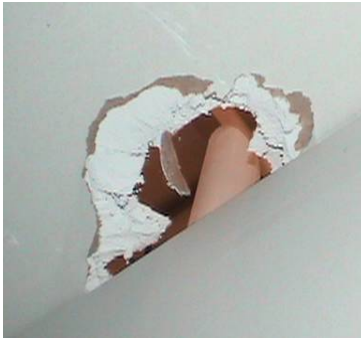
Figure 42 Vent pipe punch out
