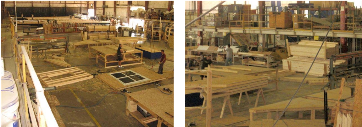
Figure 6 Dormer area before the RPI
