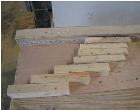
Figure 25 Fixture to cut studs to size, reducing manual measuring
