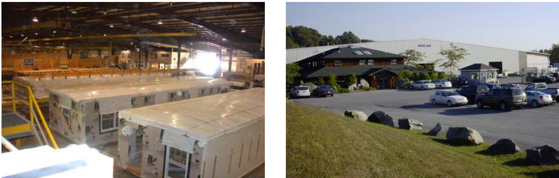
Figure 27 Chelsea's plant, interior and exterior
