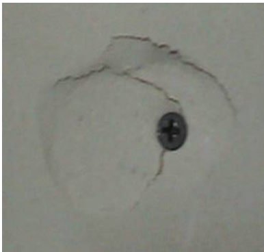
Figure 39 Hammer mark from setting screw
