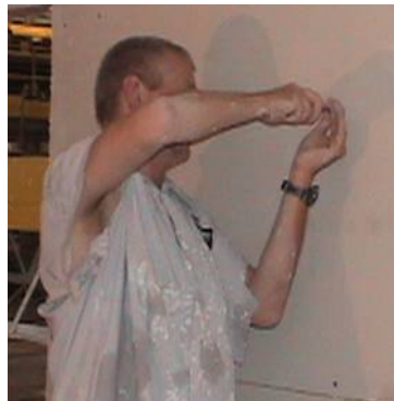
Figure 40 Taper setting screws by hand
