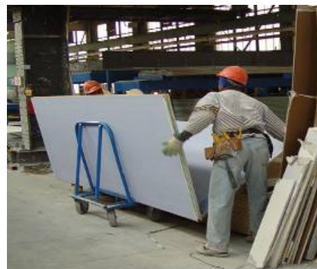
Figure 29 Loading gypsum board on a cart
