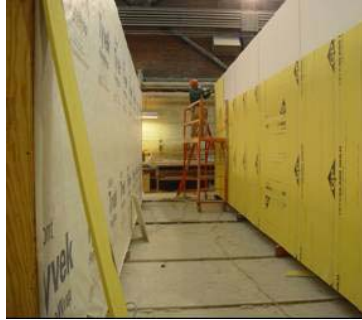
Figure 33 Installing yellow-faced gypsum board
