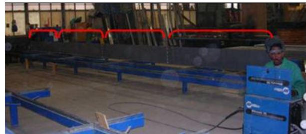
Figure 31 Welded sections of ceiling rim joist
