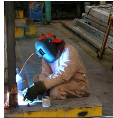
Figure 39 Welding a corner post
