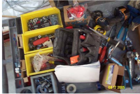
Figure 57 Cart with parts and tools in pile
