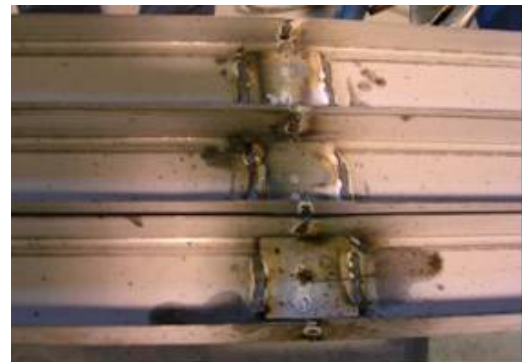
Figure 32 Welded wall track
