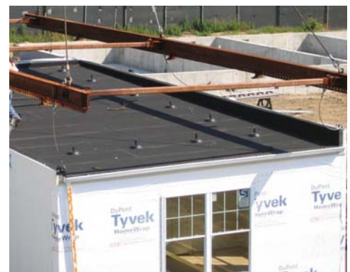
Figure 55 Triangular parapet wall
