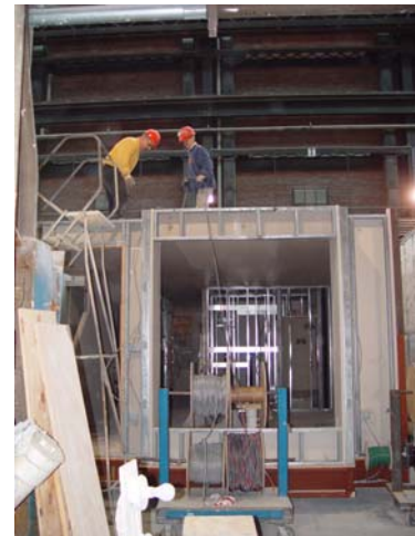
Figure 22 Working on top of a module
