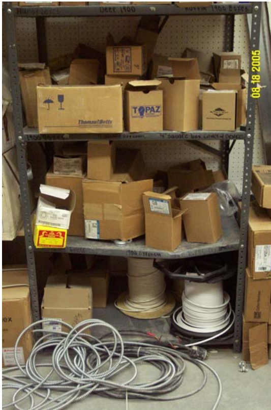
Figure 58 Mixed parts in electrical stockroom prior to the RPI event
