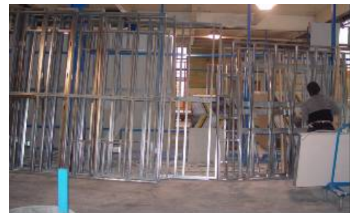
Figure 47 Wall frames ready for gypsum board
