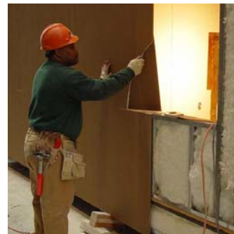
Figure 36 Trimming gypsum board
