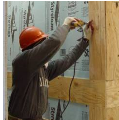
Figure 35 Installing furring strips with an electric drill
