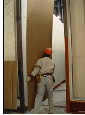
Figure 34 Installing 12 foot long gypsum board on a demising wall
