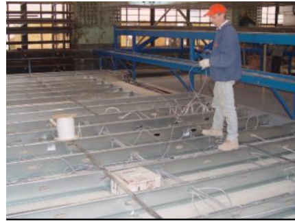
Figure 38 Wiring the ceiling on the ceiling cart
