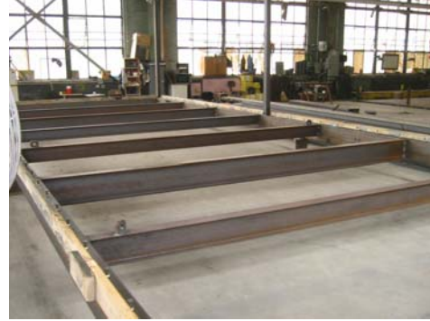
Figure 51 Floor frame for concrete floor module
