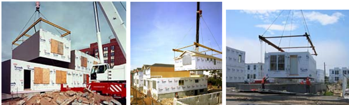
Figure 11 Capsys modules being set on three typical residential projects
