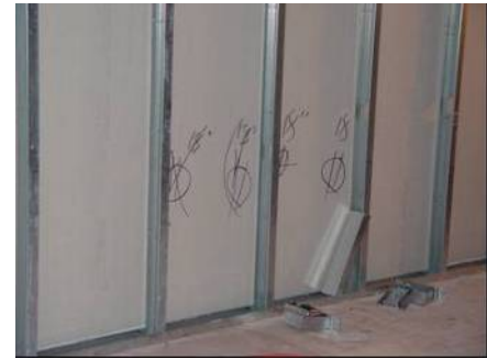
Figure 46 Relocating an electrical box
