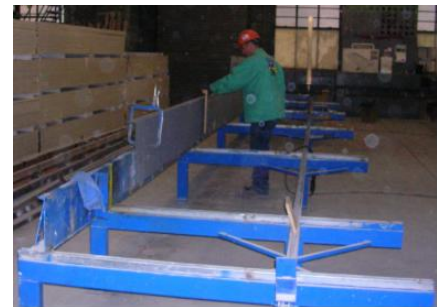
Figure 37 Placing ceiling hanger angle sections in the ceiling jig
