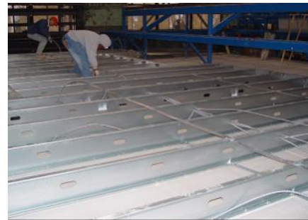
Figure 24 Wiring on the ceiling cart
