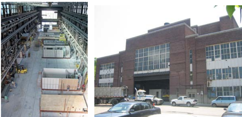
Figure 9 Capsys plant, interior and exterior
