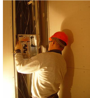
Figure 27 Installing an electrical panel
