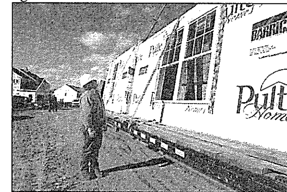
FIG. 9 SIP Walls Delivered to Building Site
