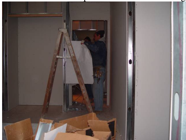
Figure 36. Electricians with framers discussing location of boxes
