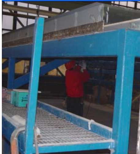
Figure 29. Operator attaching drywall onto the ceiling frame
