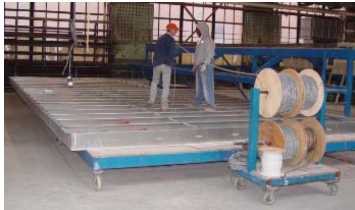
Figure 31. Wiring ceiling on ceiling cart at floor level
