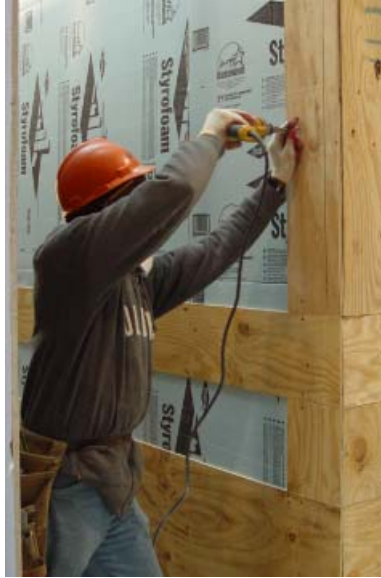
Figure 26. Manual feed drills
