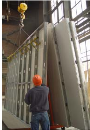
Figure 7. Lifting wall panel before set
