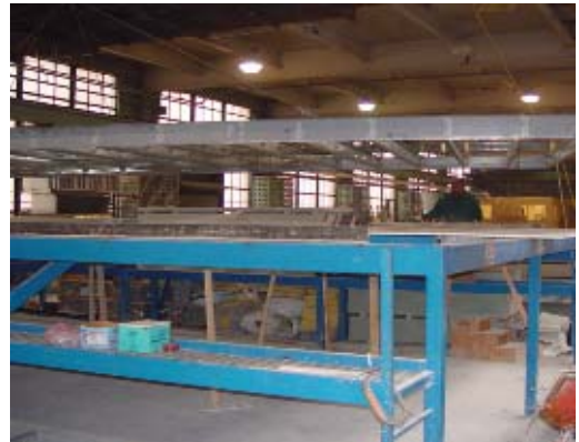
Figure 5. Positioning additional drywall
