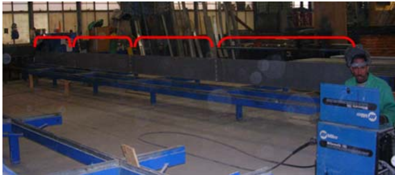
Figure 17. Ceiling rim joist is made up of 4 components welded
