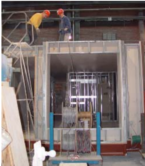
Figure 32. Electricians wiring ceiling after set on module
