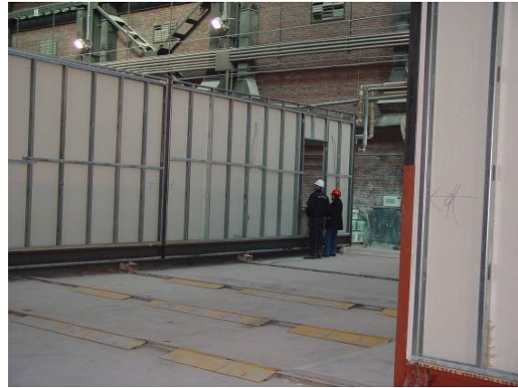
Figure 39. Wall slope and corrective trusses
