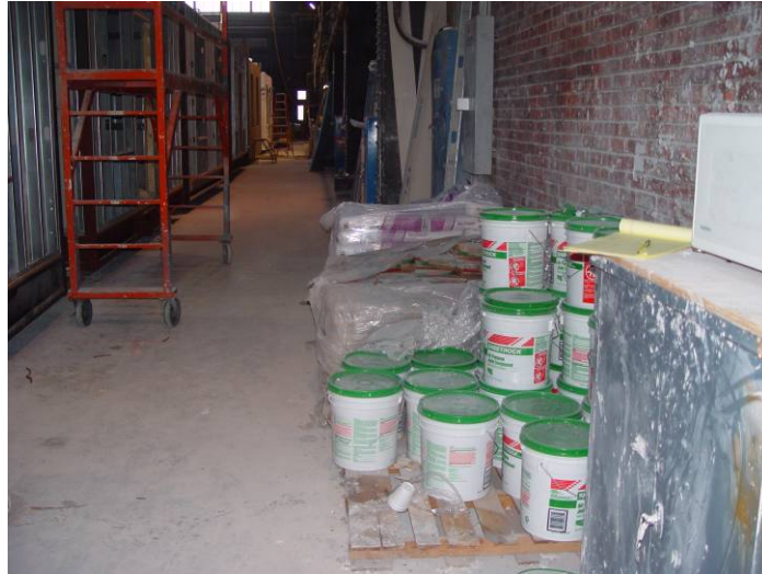
Figure 15. Mud mix station far from point of use near end of line
