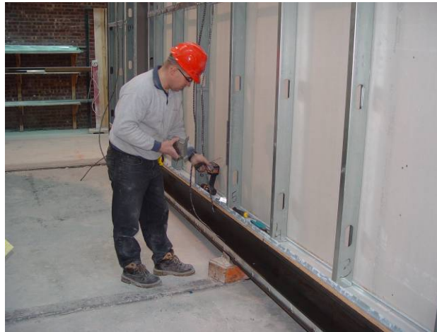
Figure 35. Installing electrical boxes after ceiling set
