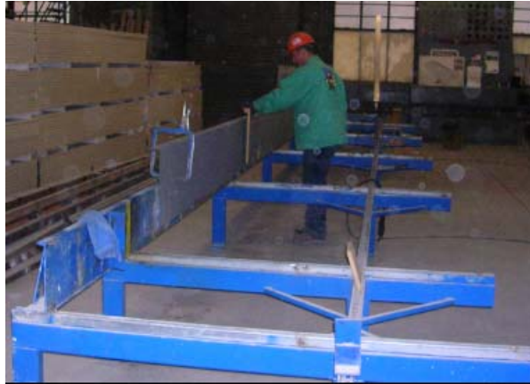
Figure 28. Operator measuring and marking location for joist hangers
