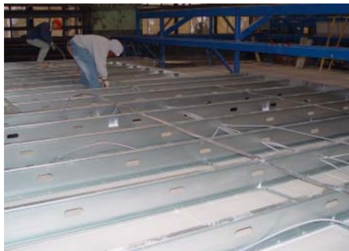
Figure 34. Pulling wires
