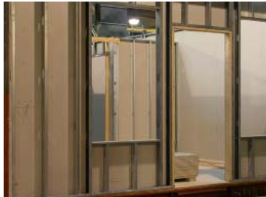
Figure 6. Window frame in wall
