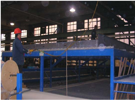
Figure 4. Re-lifting ceiling frame
