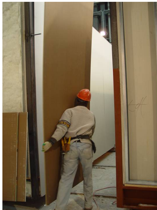
Figure 19. Installation of 12' drywall sheets
