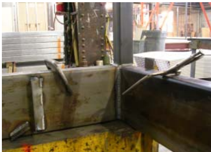
Figure 21. Floor framing- rim joist and joist hangers welded
