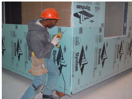
Figure 3. Installing foam sheet using screws
