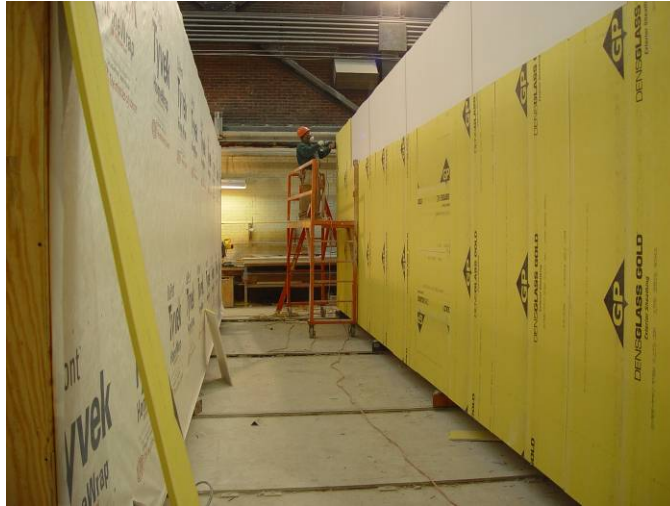
Figure 10. Operator reworking drywall
