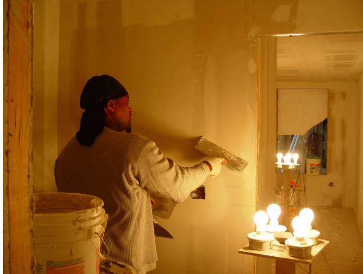
Figure 11. Drywall finishing
