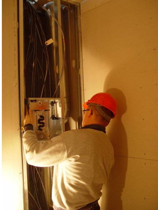
Figure 13. Electrician installing panel
