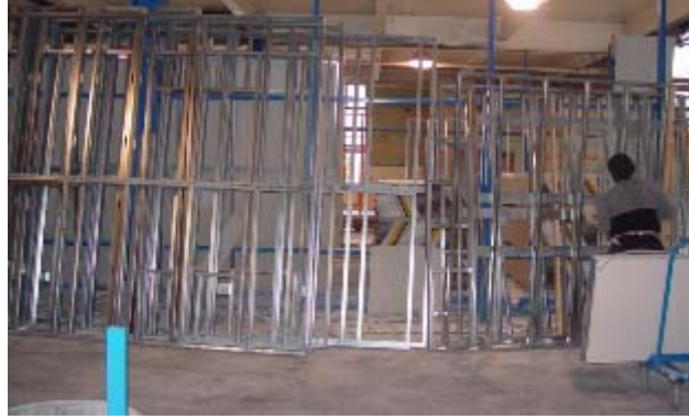
Figure 9. Labeled wall frames staged for drywall installation
