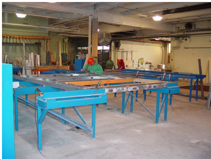
Figure 25. Wall framing using screw attachments
