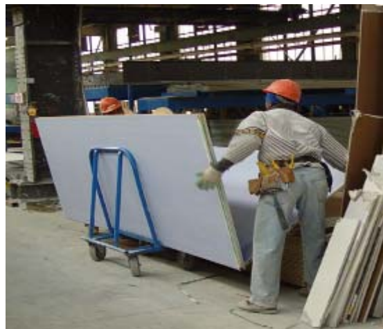
Figure 14. Operators loading drywall onto cart
