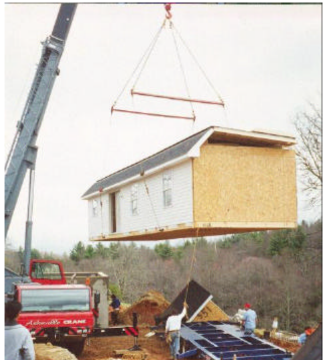
Figure 1. Setting a typical module
